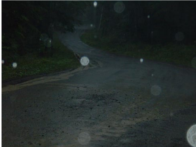
Photographs of Deer Creek Road on June 30, 2009 showing sediment entering the public road and drainage ditch from the Jackson construction site. Photo below shows runoff flowing off roadway into wetland area.
